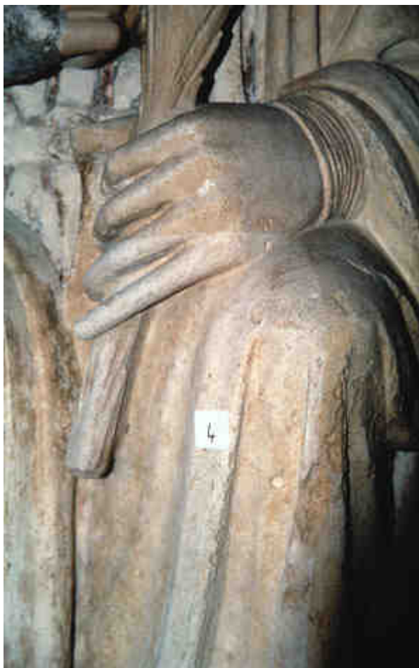
Photo 3: Attenuation of the yellow tinge caused by laser cleaning, through the application of water compresses in the lower part of the image; restoration of the central portal of the western facade of Notre-Dame Cathedral in Paris (Photo: M. Labouré).
