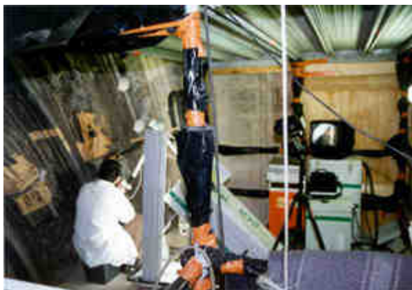
Photo 4: Interior of work zone on a laser cleaning site (restoration of the north portal of the Saint-Michel Basilica in Bordeaux (Photo: T. Vieweger).
